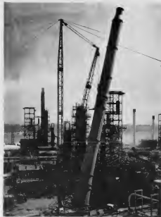
NEARLY UP, bottom must now be lined up with base. CASI CLA, ainda e base mester worde poni pareu.
